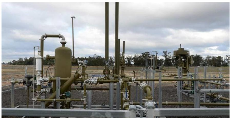
*Coal seam gas well in Queensland - photo from The Standard*
